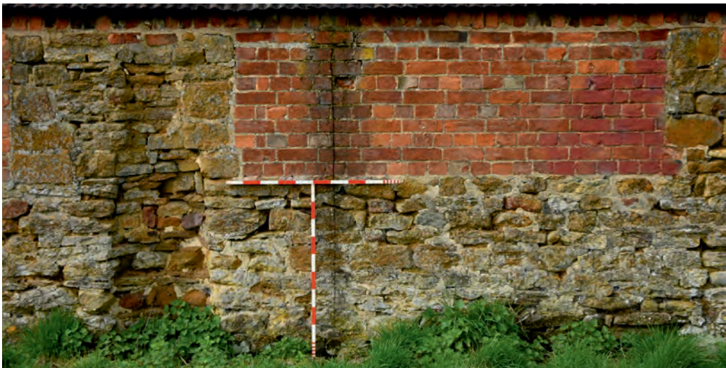
Figure 6. An example of the blocked windows. Note the 'niche' at the left of the image. (Author's photograph)
