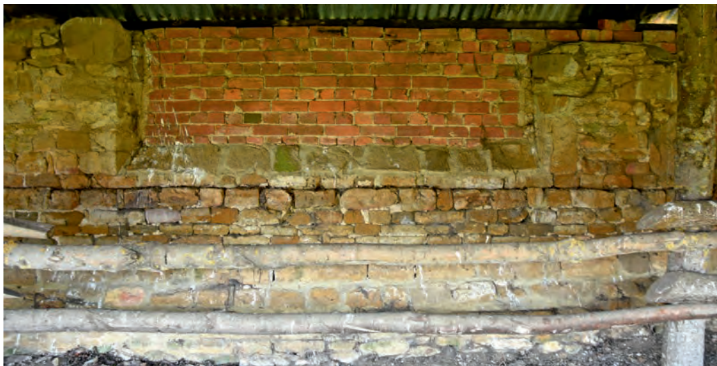
Figure 7. Internal view of one of the blocked windows (Author's photograph)
