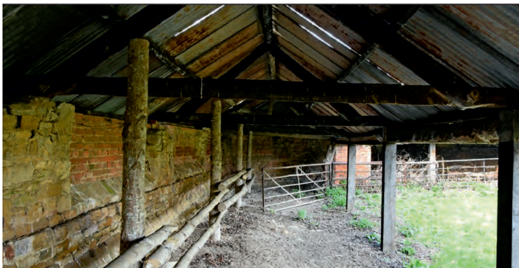
Figure 8. View along the western range, looking north (Author's photograph)
