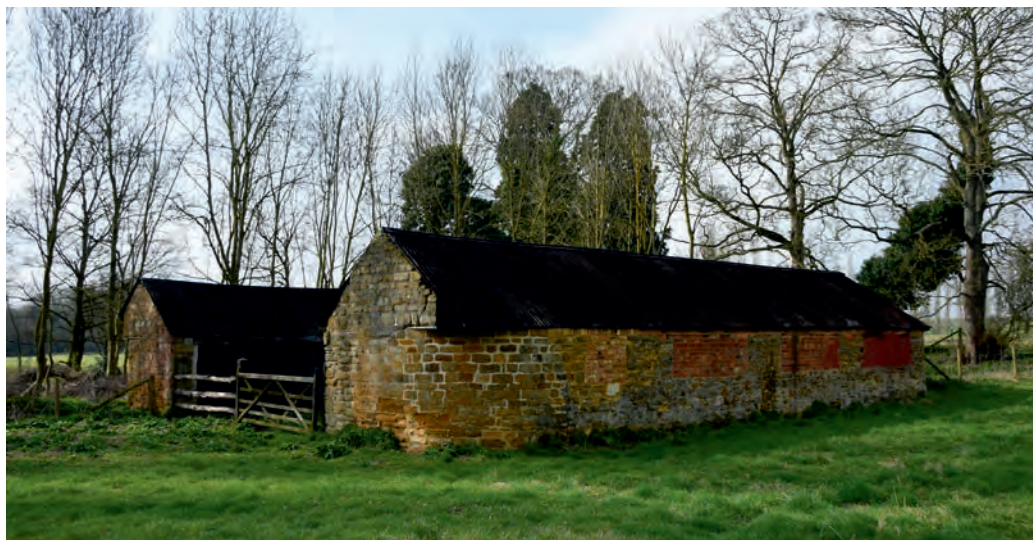
Figure 4. General view of the Ox House, looking north west (Author's photograph)
