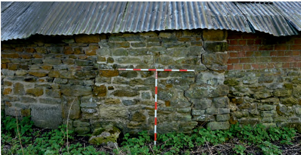
Figure 10. Blocked doorway at the centre of the north range (Author's photograph)
